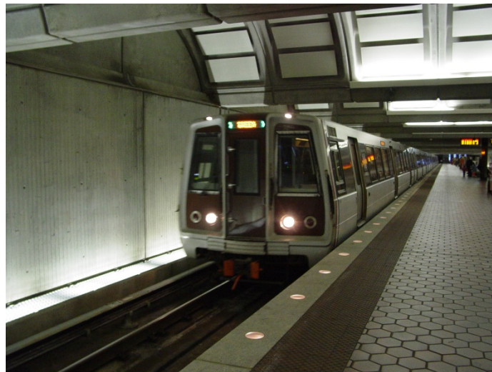
WMATA train platform showing detectable warning material behind granite edge. 4
